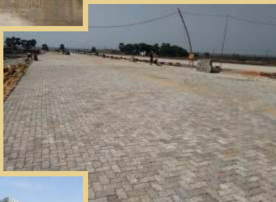
PWD Road / Industrial Park
